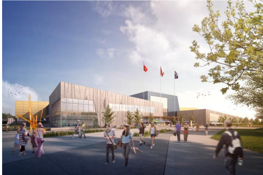
Pan Am Aquatics Centre, Southwest View – Military Trail & Morningside Ave
