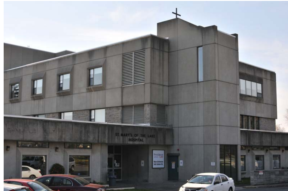
St. Mary's of the Lake Hospital Site
