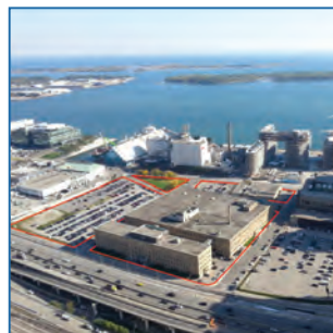
LCBO - Head office Redevelopment
