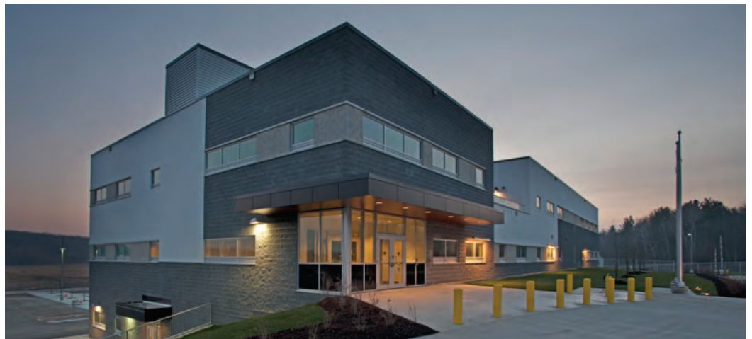
Ontario Provincial Police (OOP) Modernization Ontario Builder Award for excellence in non-residential construction to Bid, 2012
