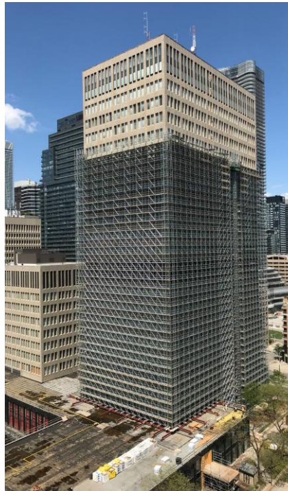
Image: Mowat Tower envelope restoration scaffolding
