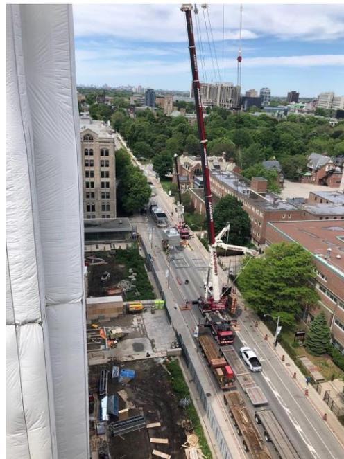
A 400-ton crane was assembled on Wellesley Street West utilizing a 90-ton crane to lift four new cooling towers onto the roof of the Ferguson building.
